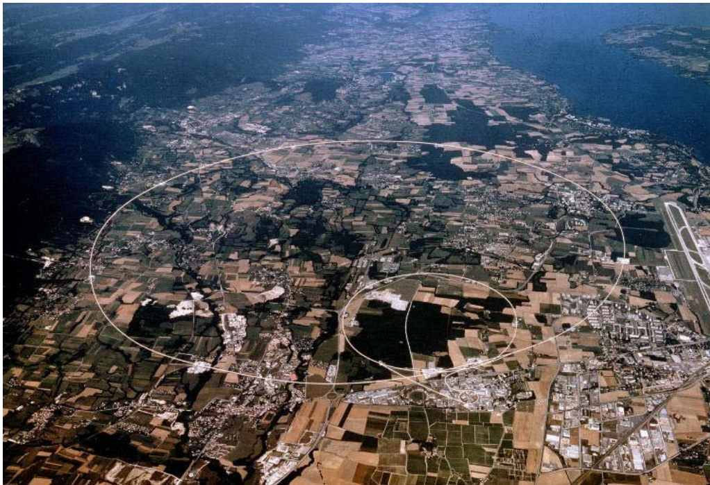
27 km circumference tunnel at CERN
